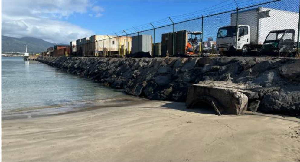
Figure 3.6 Submerged Outfall at Pier 2 (Brown and Caldwell)
