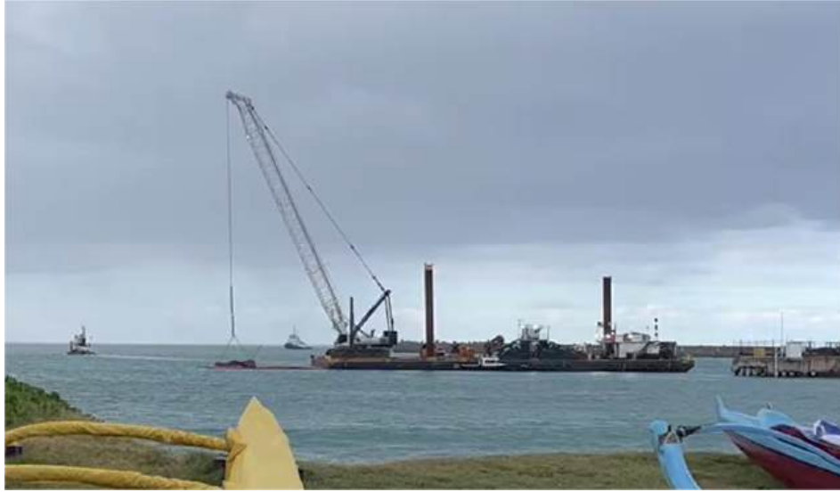
Figure 2.2 Dredging Activity March 2024 (Brown and Caldwell)
