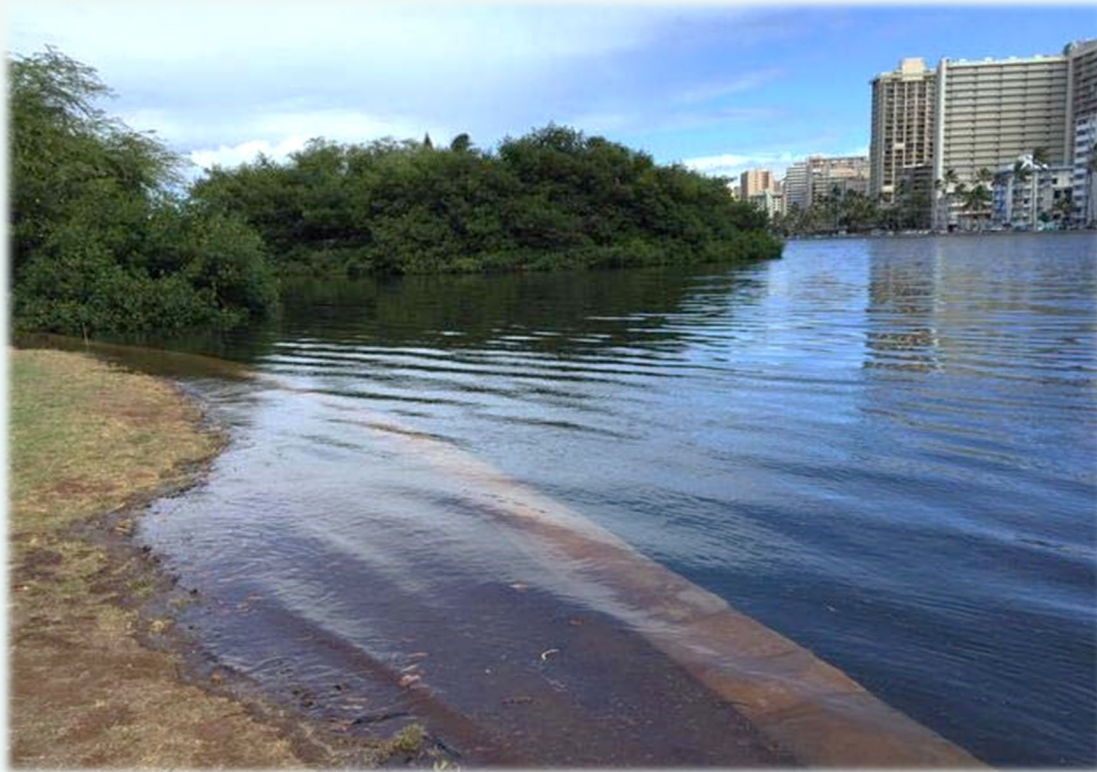
Ala Wai Canal over-topping during a King Tide Image Source: UH SOEST King Tides Project
