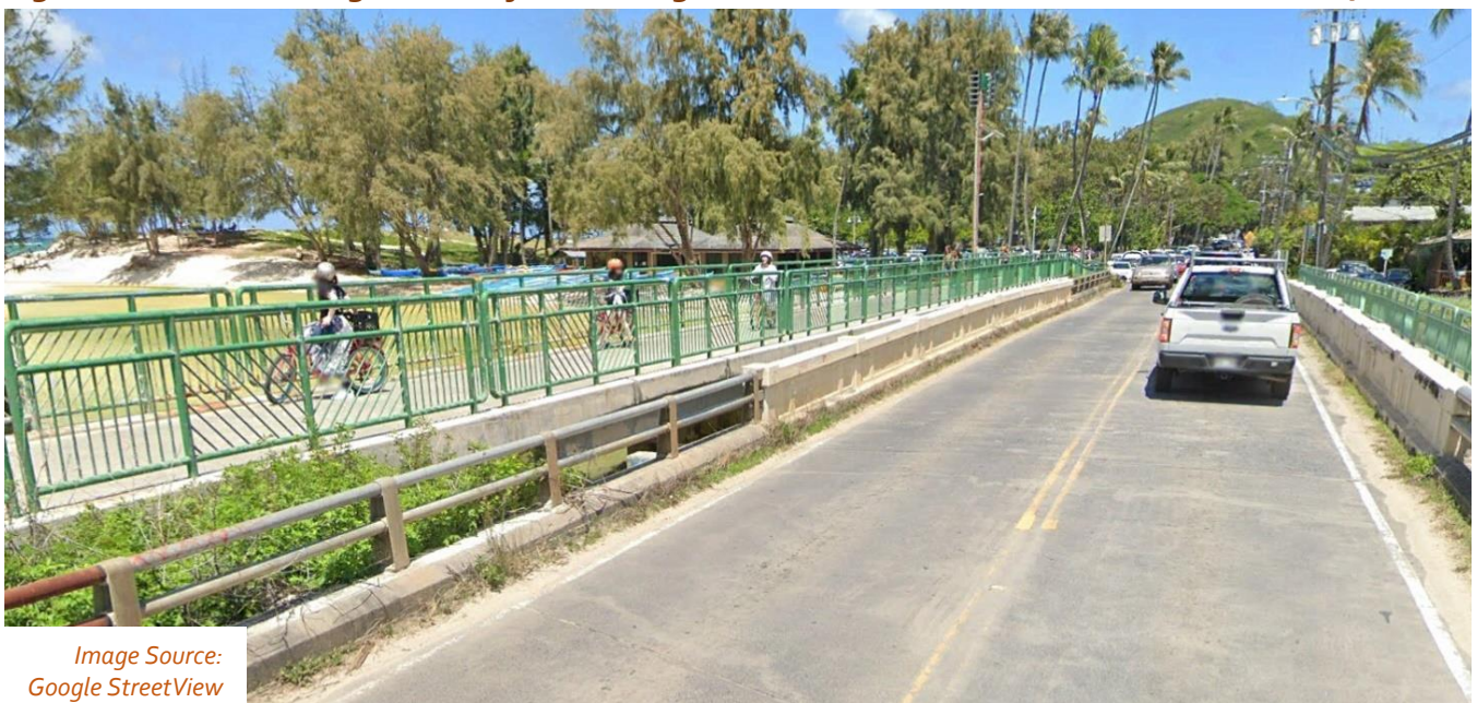
Figure 26: Historic Bridge with Adjacent Bridge Constructed for Shared-Use Path in Kailua, Oʻahu
