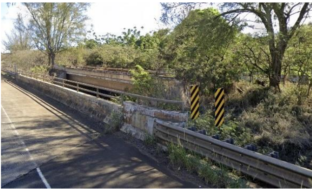
Figure 20: WMG Stream Crossing
