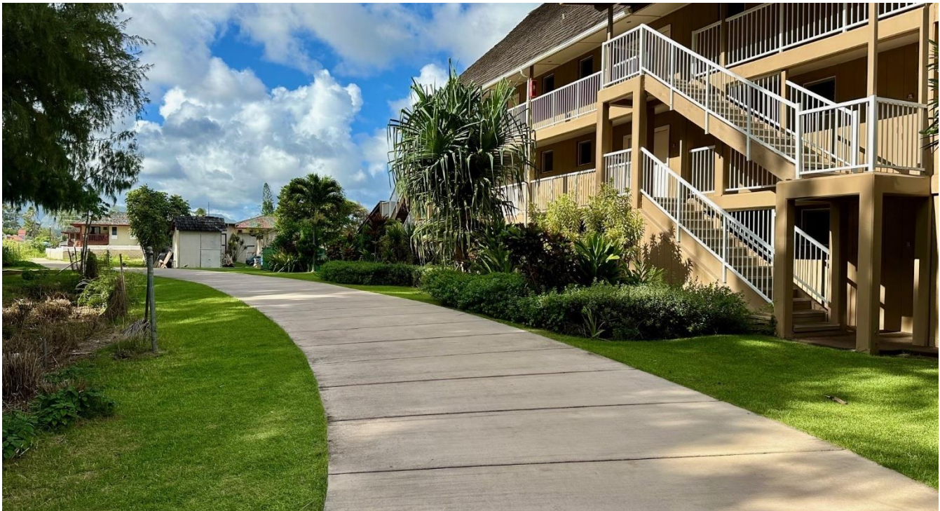
Figure 17: Ke Ala Hele Makalae Path Adjacent to Condominium
