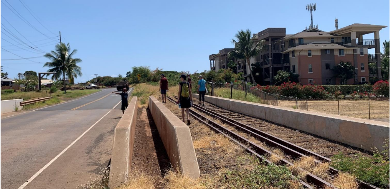
Figure 7: Segment 4 Sugar Cane Train Bridge Crossing
